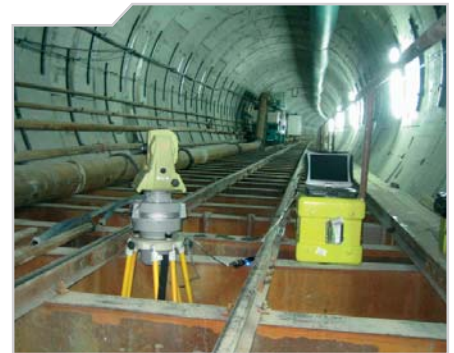
Gyro-measurement in a subway tunnel
