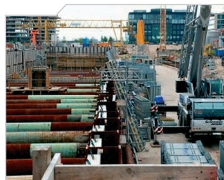
Typical application of WSM1 is for monitoring struts
