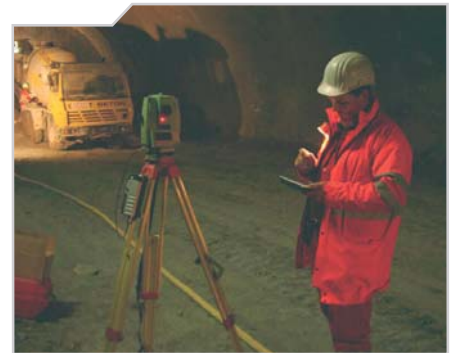
Controlling the final shotcrete layer with KRIOS
