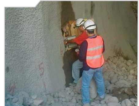
Taking readings in a measuring section
